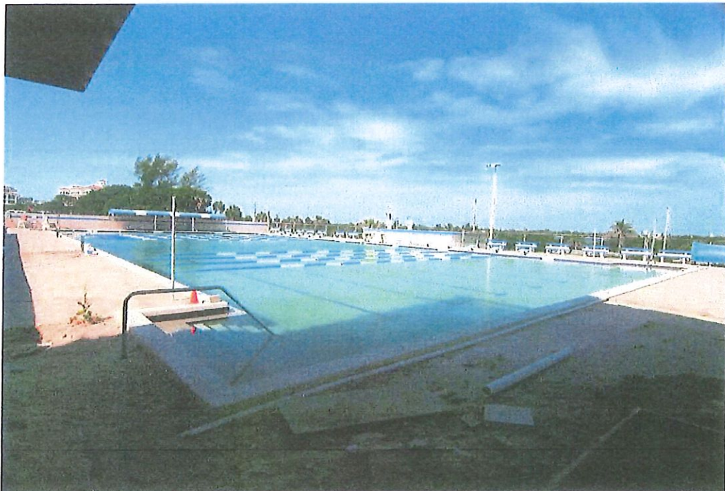
EXHIBIT 2. OVERALL VIEW OF POOL AND DECK LOOKING SOUTHWEST
