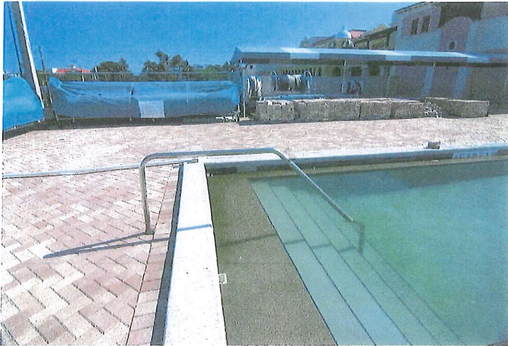
EXHIBIT 3. VIEW OF NORTHWEST AREA OF POOL
